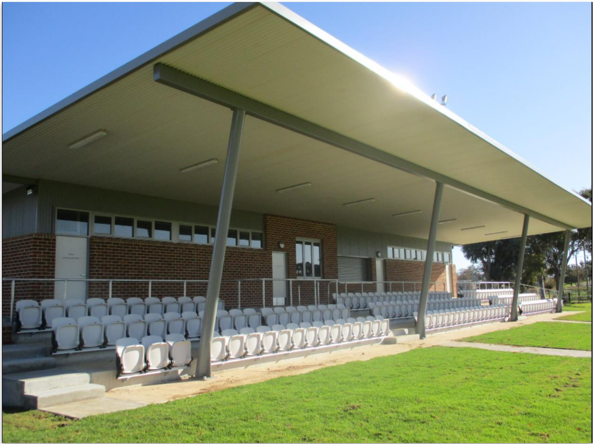
Lawson Park grandstand
