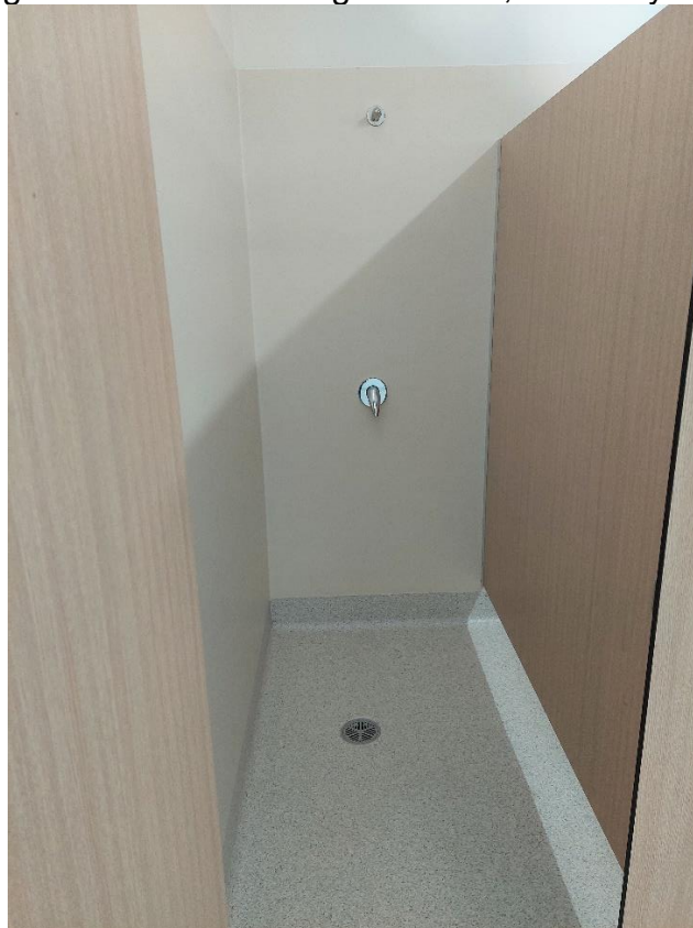
Figure 3. Photo of upgrades shower in amenities building at Quandialla Swimming Pool.
