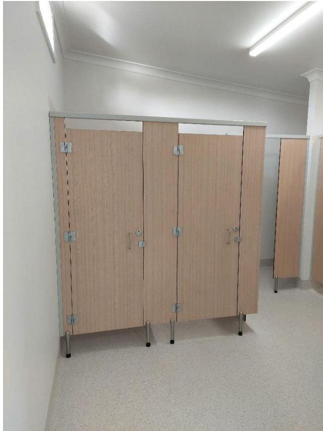
Figure 4. Photo of upgraded amenities at Quandialla Swimming Pool.
