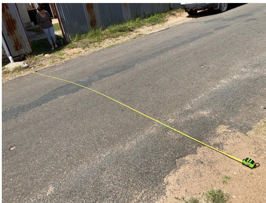
Figure 1 George Street is 6 meters wide and does not have kerb, gutter or footpaths
