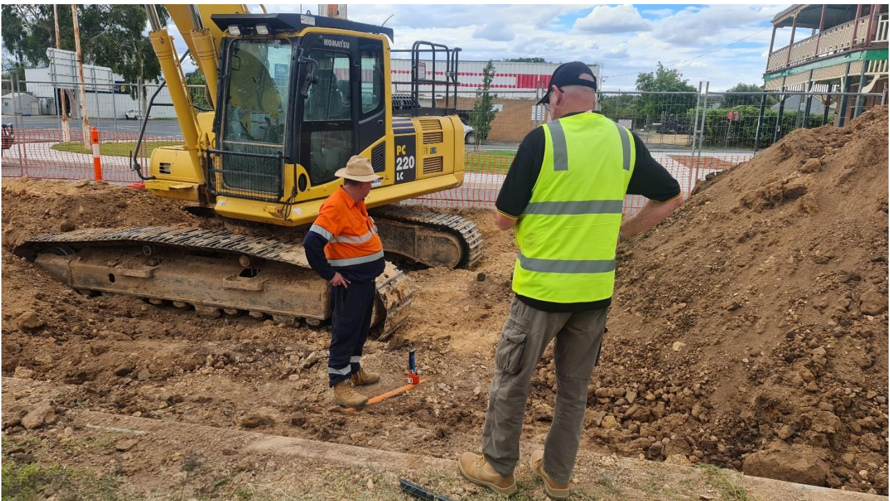
WSC determining what unknown service is at Stage 1, service not shown on DBYD or WSC GIS
