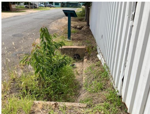
Figure 3 George Street has many trip hazards including open drains.
