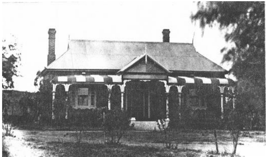
Glen Park early photo, note striped verandah roof
